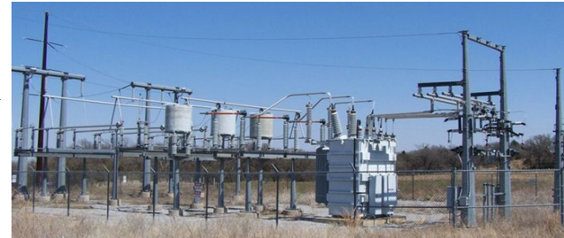
Substation 15,000V
